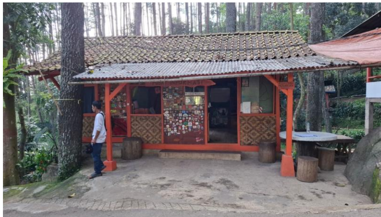
Gambar 5. 1 Kondisi Eksisting Bangunan TIC & Hiking Center
