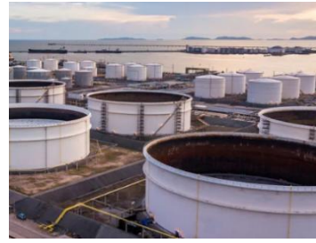
floating roof tank
