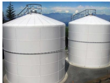
fixed roof tank
