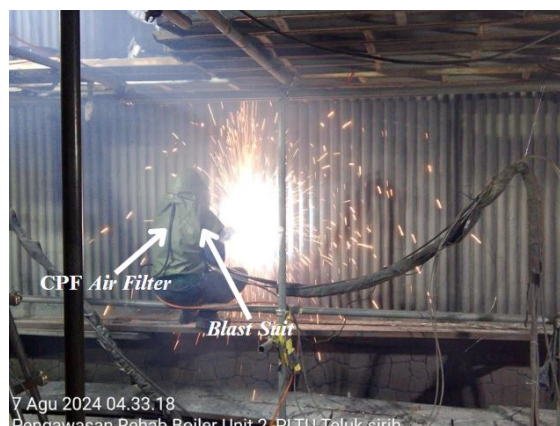
Gambar 51. Proses metal coating
