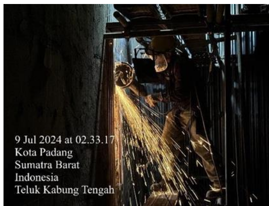
Gambar 35. Cutting tube exiting
