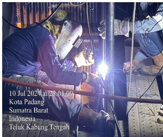
Gambar 41. Proses tack welding
