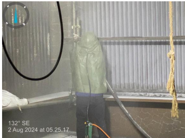
Gambar 50. Proses sanblasting
