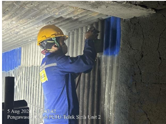
Gambar 57. Proses ceramic coating
