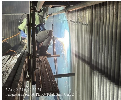
Gambar 52. Proses metal coating
