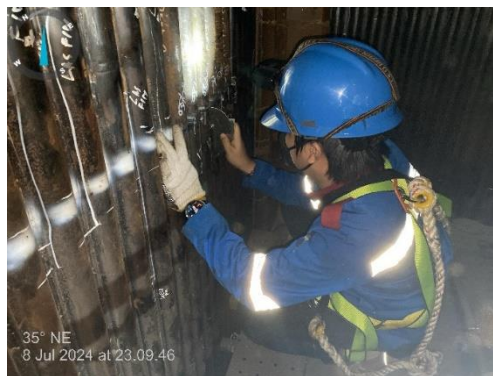
Gambar 62. Mengukur capping
