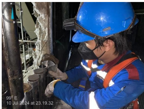
Gambar 63. Mengukur V-grove
