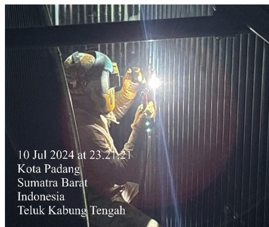
Gambar 43. Proses Welding Tube GTAW
