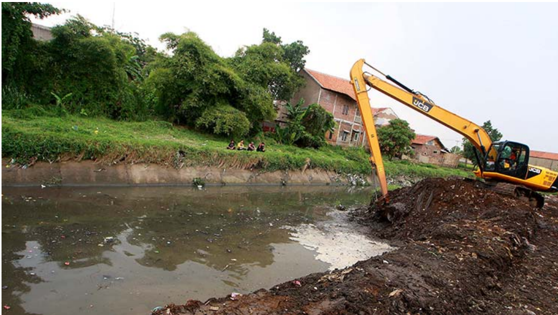
Figure 2. Dredging Sedimentation on Normalization Watershed Cikapundung project in 2015
