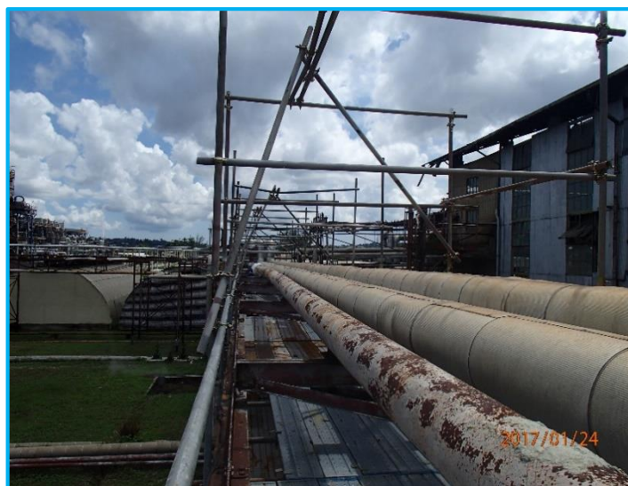
Gambar 1.1 Sistem perpipaan steam 17 bar
