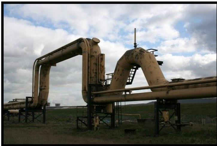
Gambar 2.19 *Expantion Loop*
