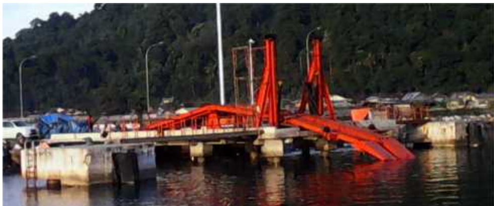
Gambar 4.5 Proses Unloading Ramp Gate Door
